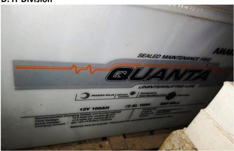
100AH Lead-Acid SMF battery **AMARON- QUANTA-12V-100AH SMF--- 10 nos**With rack
